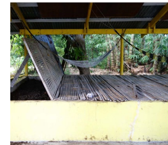
Example of vermicomposting installation (Source: EAWAG)
