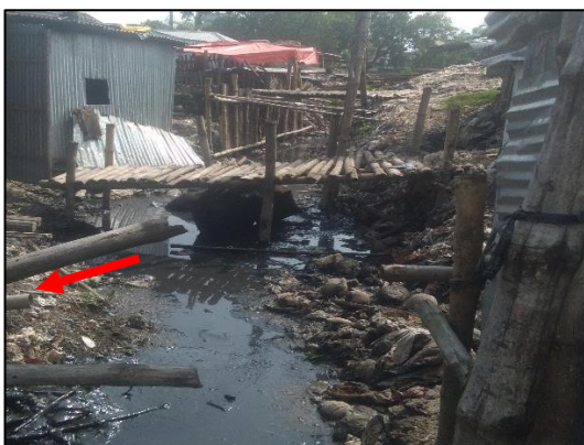
Septic tank connected to a nearby water body
