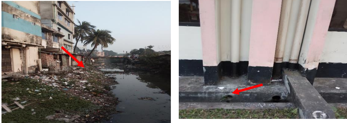
Figure 5: Containment technologies and their connections in Patuakhali. Left: Toilet Pit open to a nearby water body, Right: Toilet pipe connected to open environment (Source: Feasibility study 2020-21/DPHE )
