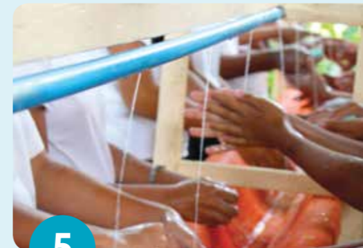
5. Punched water pipes reduce cost and water consumption
