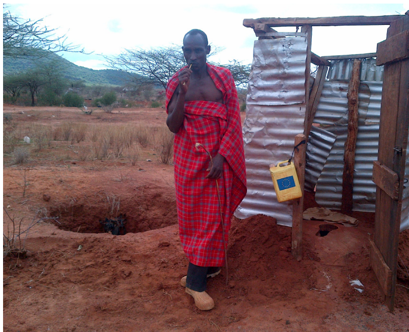
Community member in Arumrum, Isiolo district, with his latrine (dome shaped slab and super-structure made from locally available materials) and deep rubbish pit for household waste.
