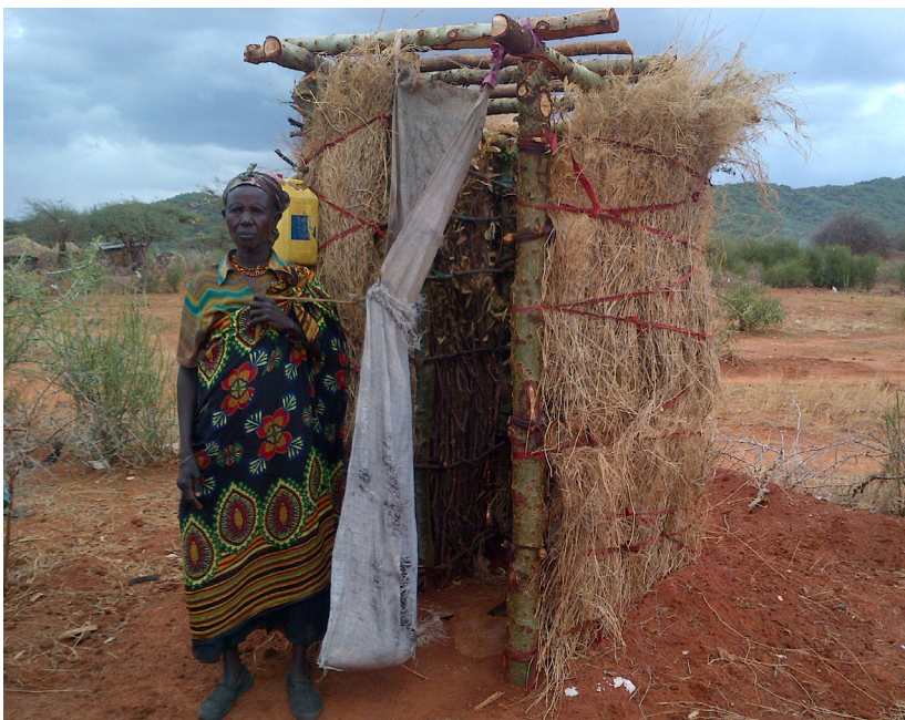
Locally constructed household latrine in Arumrum community, Isiolo district
