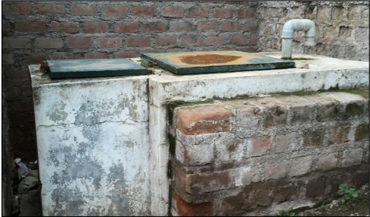
Figure 4: Inspection point 3 - Pressure reduction shaft
