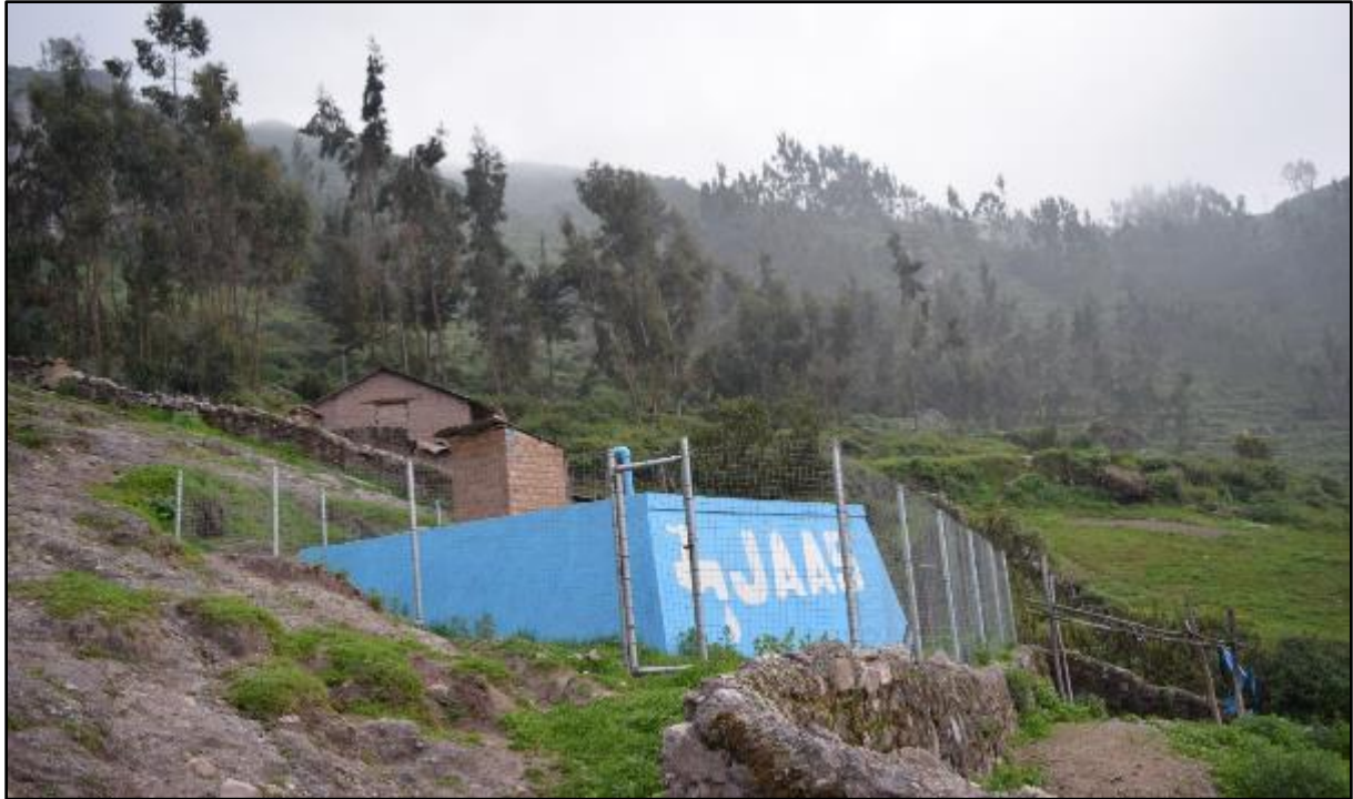
Figure 2: Inspection point 1 - Main water tank
