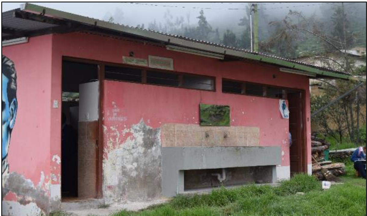
Figure 7: Inspection point 6 - School toilets
