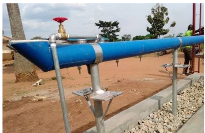
FIGURE 7 // LEFT: WASHaLOT main pipe. LEFT BELOW: Stainless steel water outlets (nozzles) (Source: photos by S. Semiyaga, 2021) FIGURE 8 // TOP: Manual refill (Source: GIZ Sanitation for Millions, 2020) FIGURE 9 // BELOW: WASHaLOT with water connection (Source: WatSSUP, 2020)
