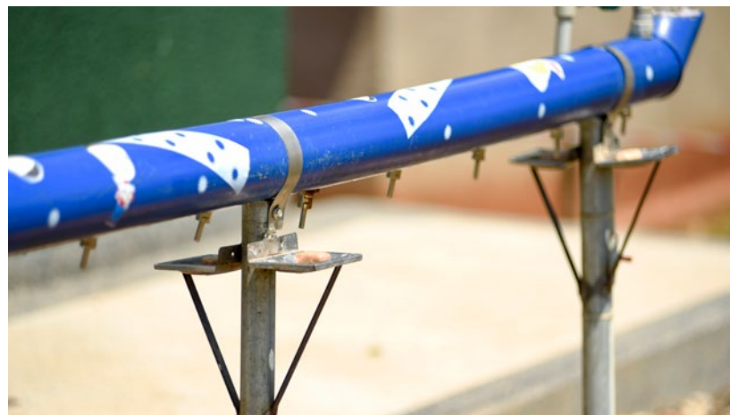
FIGURE 10 // TOP: Design for WASHaLOT stands and the stainless steel soap holders (Source: GIZ Sanitation for Millions, illustrations by D. Egessa, 2020).
