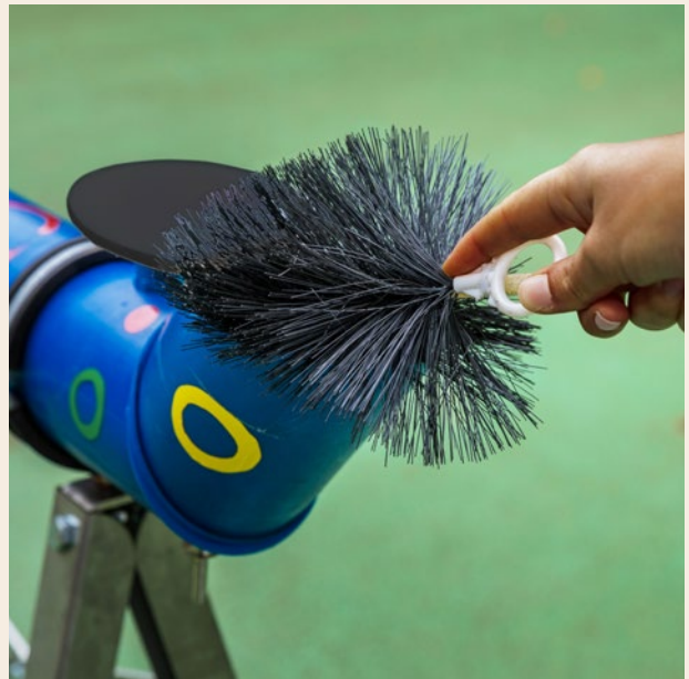
FIGURE 27 // TOP: Cleaning inside of the WASHaLOT with a brush (Source: GIZ Fit for School, photo by David Weyand, 2020) FIGURE 28 // LEFT: Examples of algae proliferation and mineral deposits due to poor maintenance (Source: photo by S. Samiyaga, 2021)
