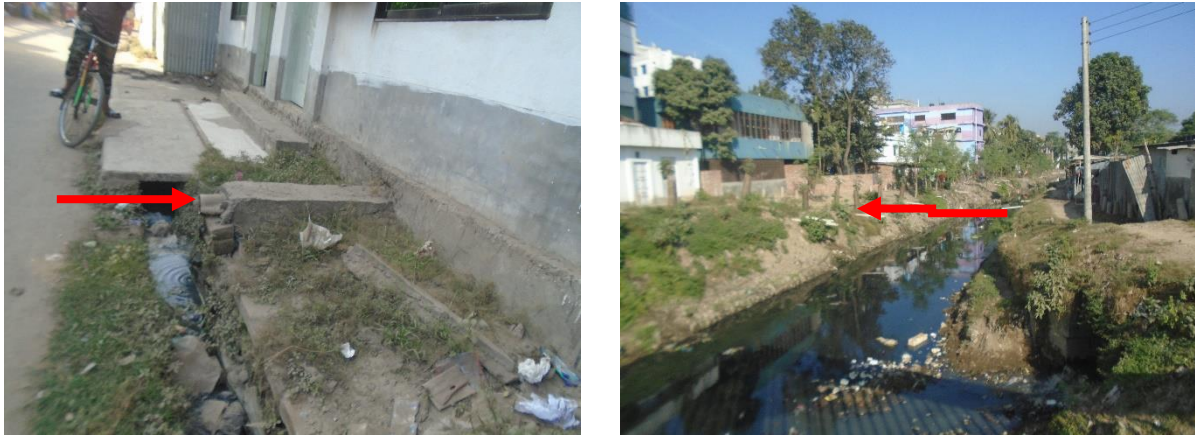
Figure 6: Containment technologies and their connections in Dinajpur. Left: Septic tank connected to the nearby water body. Right: Toilet pipe connected to open drain. (Source: Feasibility study 2020-21/DPHE).
