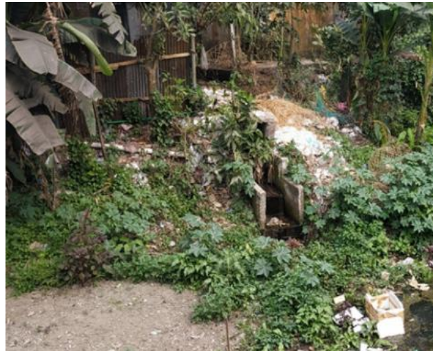
Figure 6: Containment technologies and their connections in Lakshmipur. Left: Toilet pit open to a nearby water body, Right: Toilet pipe connected to open environment (Source: Feasibility study 2020-21/DPHE ).
