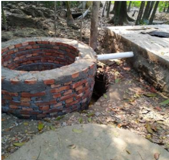
Figure 6: Containment technologies and their connections in Lakshmipur. Left: Toilet pit open to a nearby water body, Right: Toilet pipe connected to open environment (Source: Feasibility study 2020-21/DPHE ).
