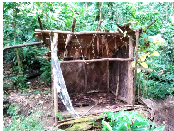
Figure 1: Typical non-compliant pit toilets (“bush toilet”) in Penama schools
