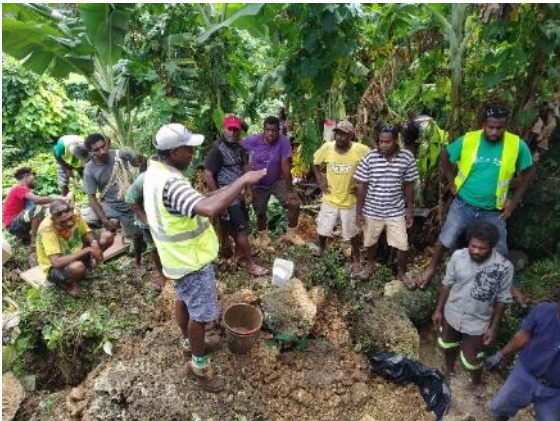
Figure 7: Spring box construction #2
