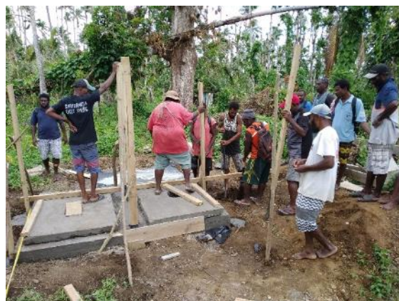
Figure 11: VIP superstructure construction
