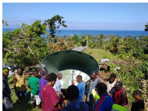
Figure 6: Storage tank installation
