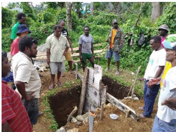
Figure 10: VIP pit construction
