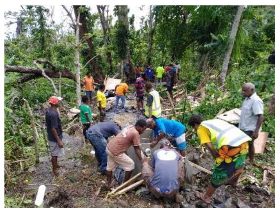
Figure 5: Spring box construction #1
