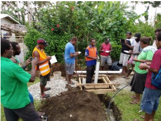
Figure 8: Tapstand installation
