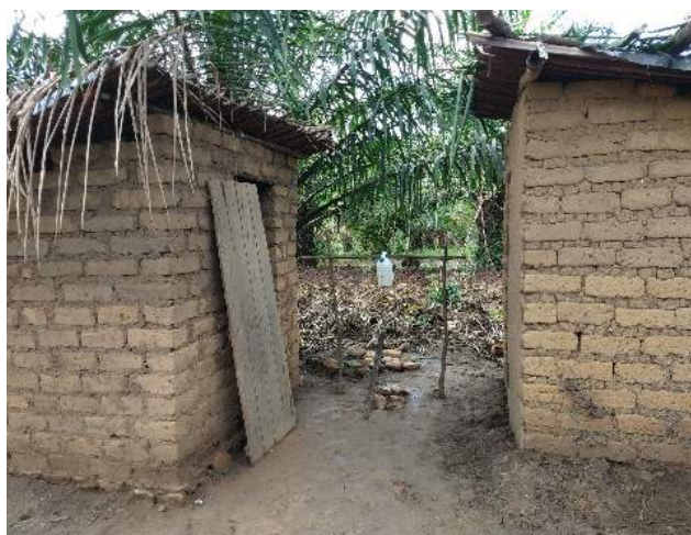
Two Akasuga latrine superstructures facing each other
