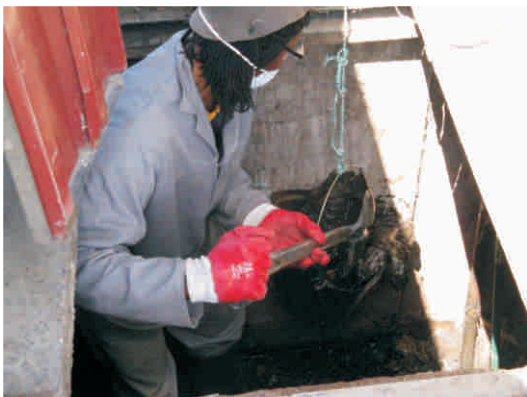
Figure 23 : Manual emptying of chambers
