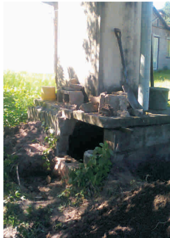
Figure 32: Many latrines are poorly designed for later emptying
