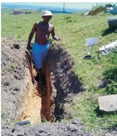
Figure 24 : On-site deep burial of sludge
