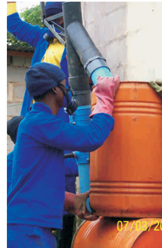
Figure 33: Using specialised tools to extract wet sludge from septic tanks
