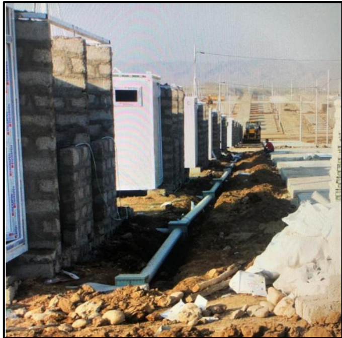
Figure 6 - Collection pipes from individual toilets (Source: Duhok Governorate, 2021)
