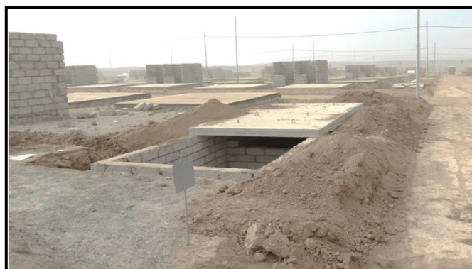
Figure 7 - Kabarto 1 Blackwater Containment, 1 of the total of 150. (Source: Duhok Governorate, 2021)
