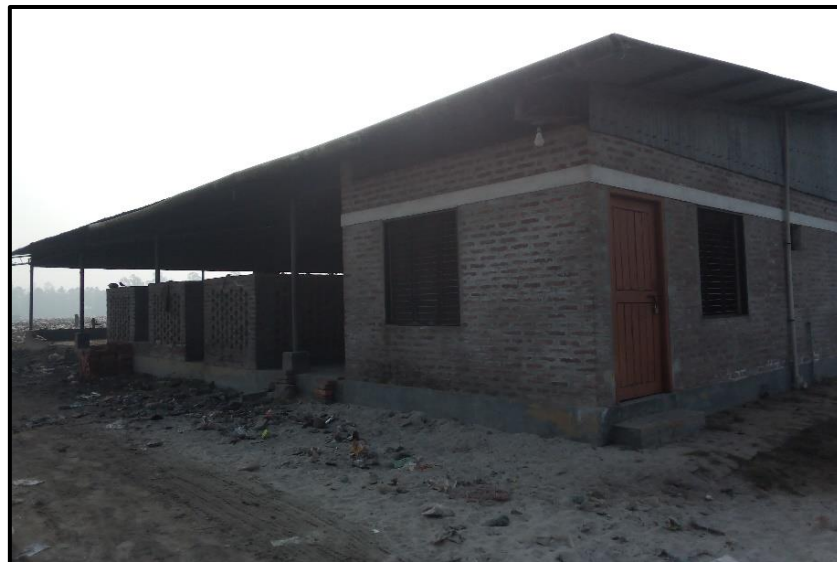
Figure 8: Faecal Sludge Treatment Plant, Sirajganj (Source: Feasibility study 2020-21/DPHE).
