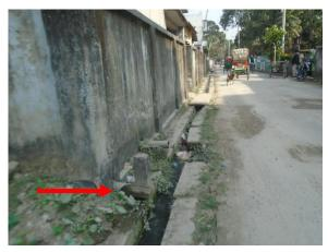
Figure 6: Containment technologies and their connections in Nilphamari. Left: Septic tank connected to the nearby water body. Right: Toilet pipe connected to open drain. (Source: Feasibility study 2020-21/DPHE).
