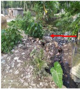
Figure 6: Containment technologies and their connections in Naogaon. Left: Septic tank connected to the nearby water body. Right: Toilet pipe connected to open drain. (Source: Feasibility study 2020-21/DPHE).
