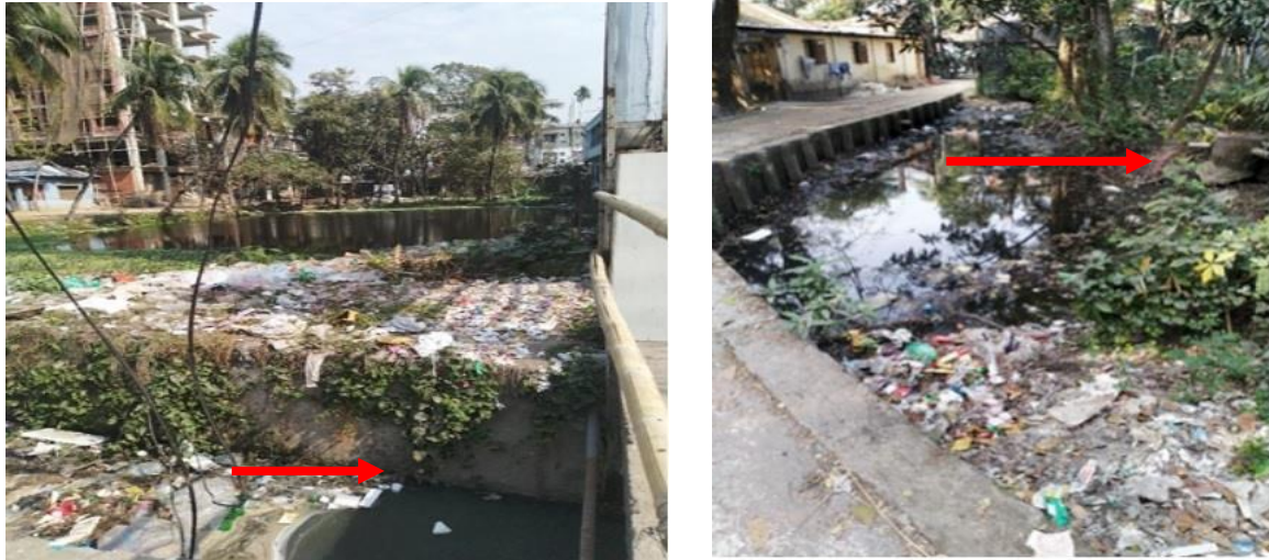
Figure 6: Containment technologies and their connections in Noakhali. Left: Septic tank connected to the nearby water body. Right: Toilet pipe connected to open drain (Source: Feasibility study 2020-21/DPHE).
