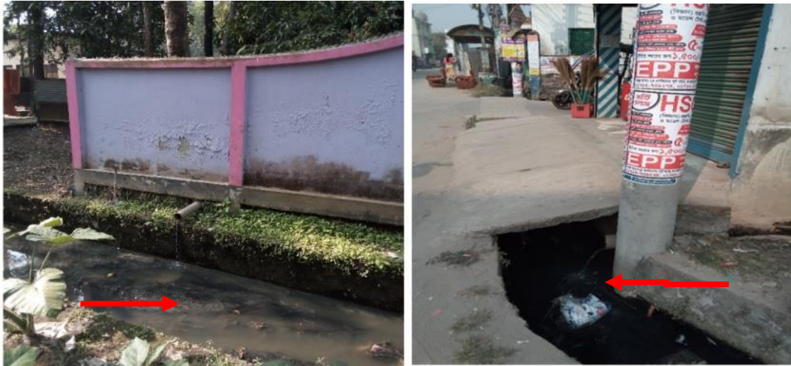
Figure 6: Containment technologies and their connections in Bogra. Left: Septic tank connected to a nearby water body. Right: Toilet pipe connected to open drain (Source: Feasibility study 2020-21/DPHE).
