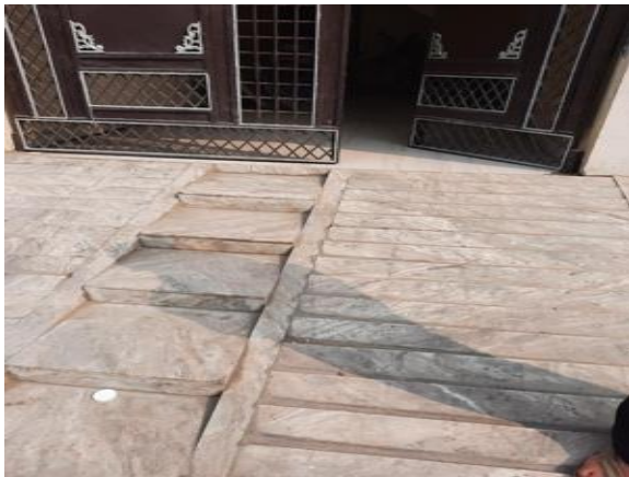
Figure 8: Fully lined tank without access-hole (Source: Aparna/NIUA/ 2020).
