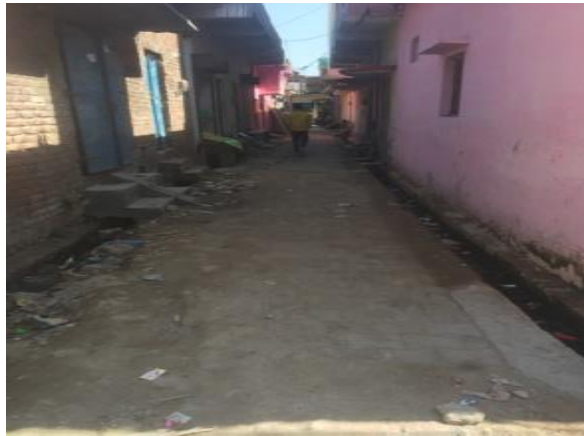
Figure 5: Grey water discharge into open drains (Source: Aparna/NIUA/2021).
