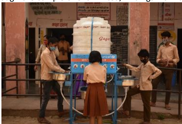
Figure 56: Children using COVID sensitive group handwashing facility installed in a school
