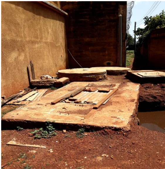
Figure 8: Image of septic tank at Tamale central prisons (CRS, 2021c)
