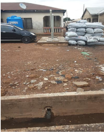
Figure 37: Septic tank connected to drain
