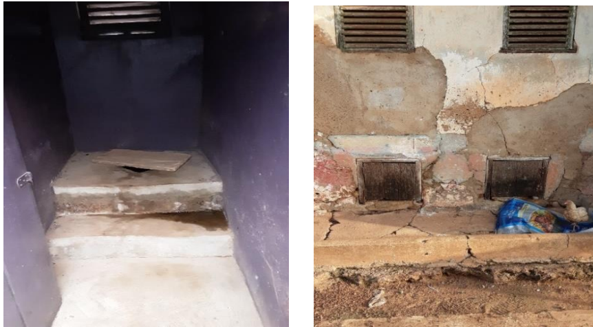
Figure 5: Images of Bucket/Pan latrine in GTA
