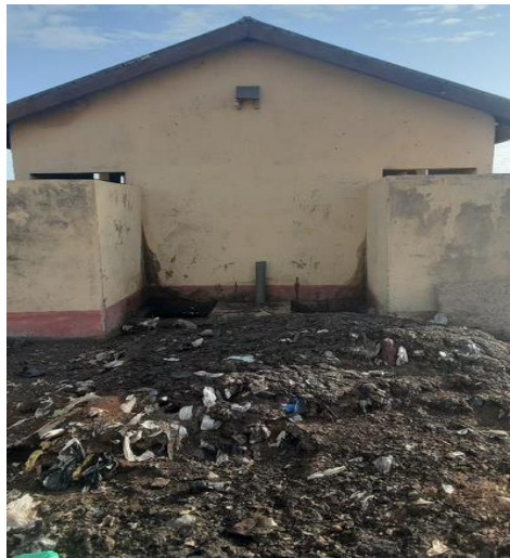
Figure 45: Exposed FS at public toilet site
