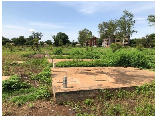
Figure 6: Image of SSNIT centralised septic tanks
