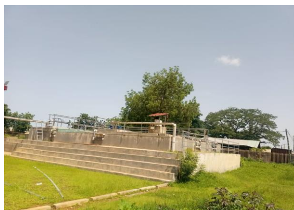
Figure 14: Image of treatment plant at Tamale Teaching hospital
