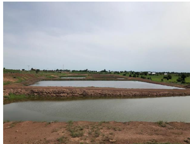
Figure 19: Newly constructed maturation pond
