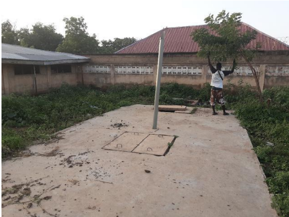
Figure 42: A public toilet in good condition
