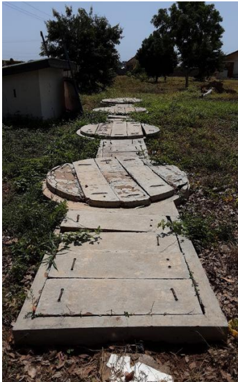
Figure 46: Centralised Septic tank at the SOS Children's home
