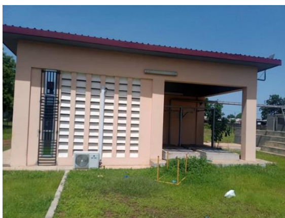
Figure 13: Control room of the treatment plant
