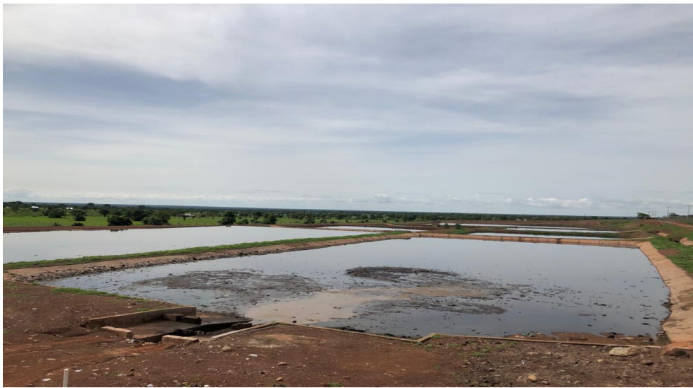
Figure 17: Gbalahi Waste Stabilization Pond
