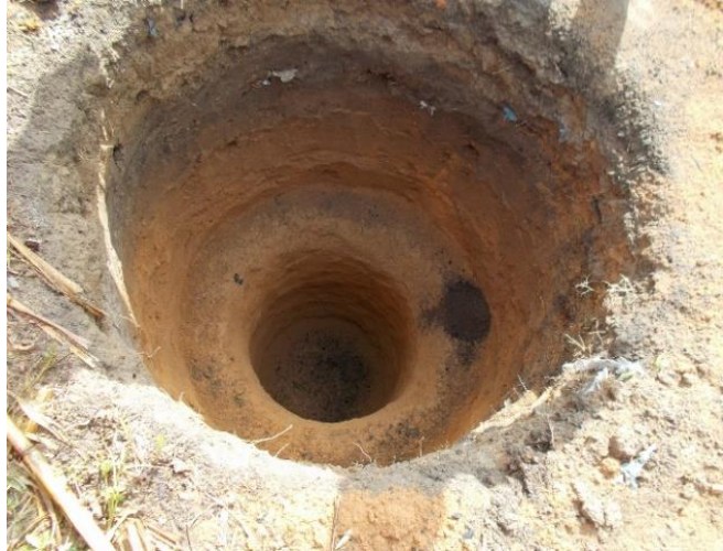
1. Site selection and pit digging
