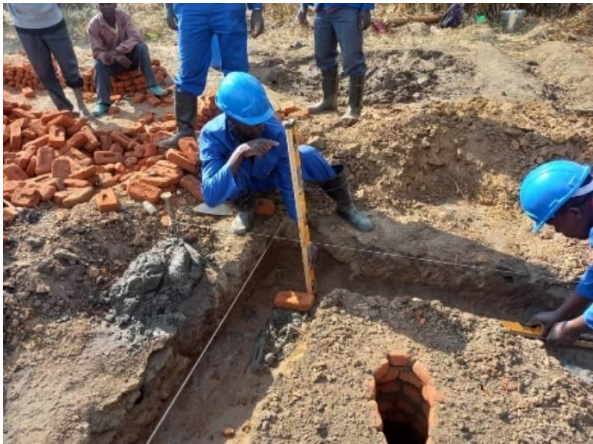
3. Finishing top part & drop-hole
