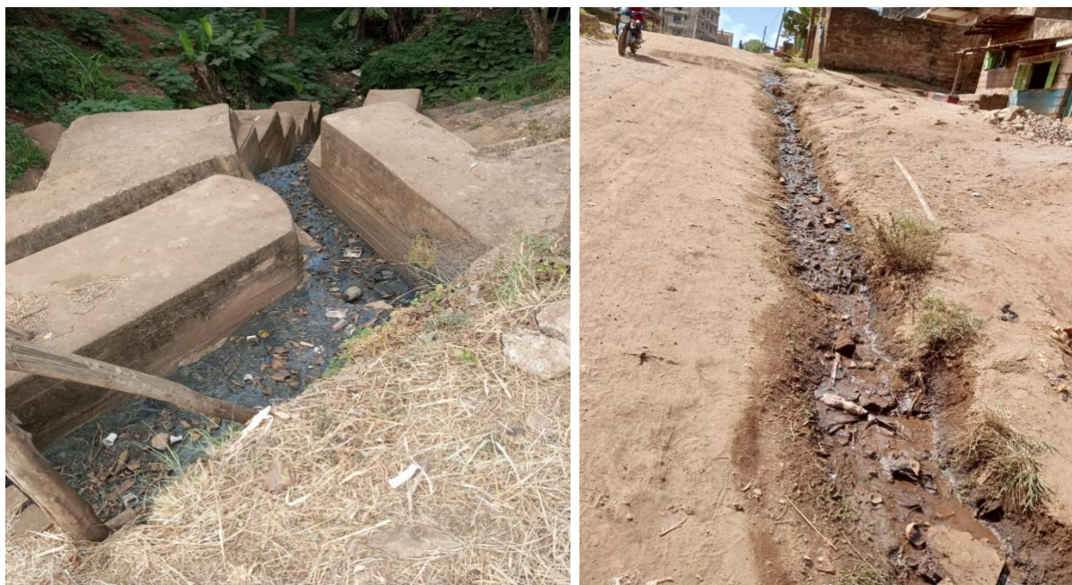
Figure 5: An open drain with raw sewage flowing to a river and households discharging wastewater to the roadside.
