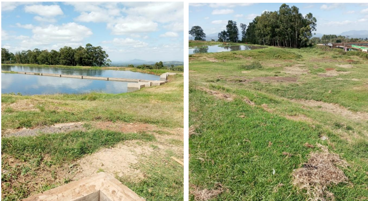
Figure 4: Images taken at Gakoromone Sewer Treatment Plant on June 2022.
