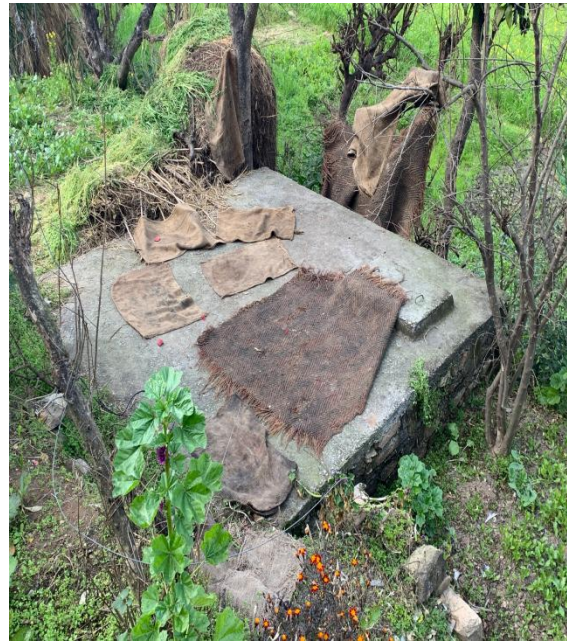
Figure 4: Lined tanks with impermeable walls and open bottom having no outlet (Source: Laila/NIUA/2020).
