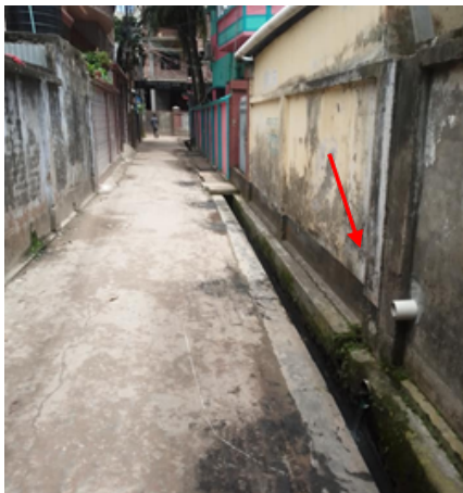
Figure 6 : Containment technologies and their connections in Chandpur Left: Toilet Pit open to a nearby water body, Right: Toilet pipe connected to open environment (Source: Feasibility study 2020-21/DPHE).
