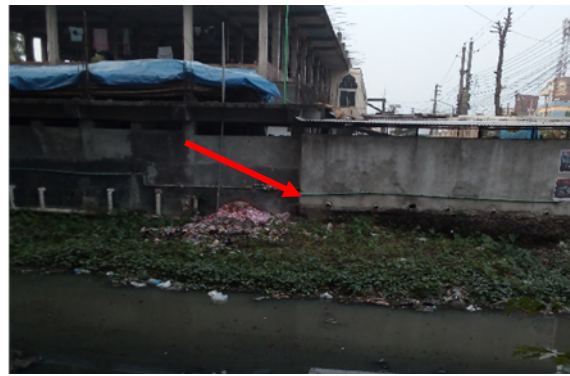
Figure 6: Containment technologies and their connections in Barishal. Left: Toilet Pit open to a nearby water body, Right: Toilet pipe connected to open environment (Source: Feasibility study 2020-21/DPHE).
