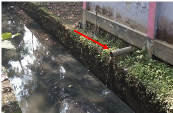
Figure 6: Containment technologies and their connections in Barishal. Left: Toilet Pit open to a nearby water body, Right: Toilet pipe connected to open environment (Source: Feasibility study 2020-21/DPHE).
