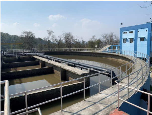
Figure 3: STP with circular SBR tank: Motharawala STP 20 MLD Dehradun (Source: Laila/NIUA/2020).
