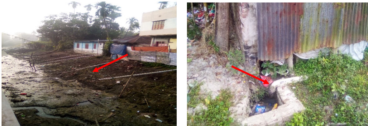
Figure 6 : Containment technologies and their connections in Bhola. Left: Septic tank connected to nearby water body. Right: Toilet pipe connected to open drain (Source: Feasibility study 2020-21/DPHE ).
