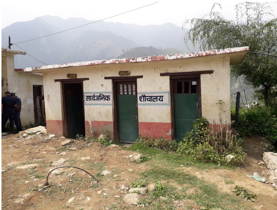
Figure 8: Public Toilet at Badimalika Municipality.
