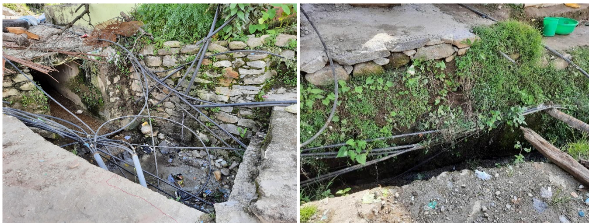
Figure 15: Storm Water Drain in urban area of Badimalika Municipality.
