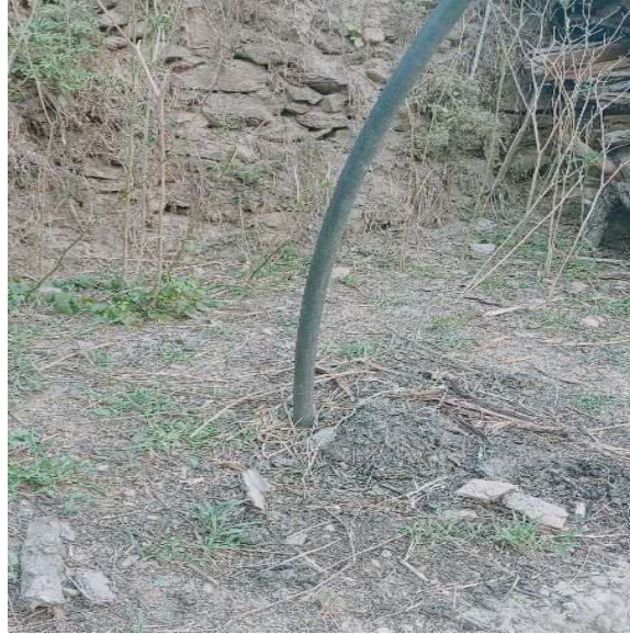
Figure 8: Top view of unlined pit with an exhaust pipe.
