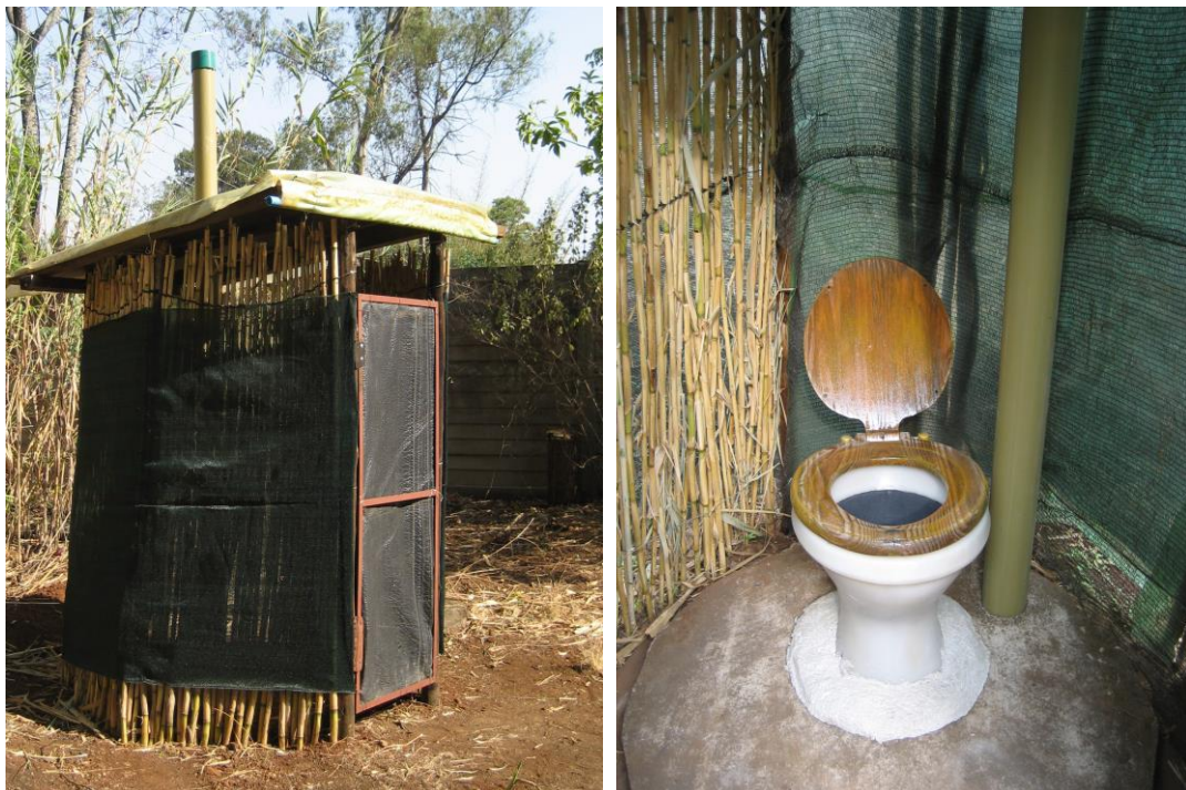
The completed toilet fitted with pedestal and screened vent pipe
