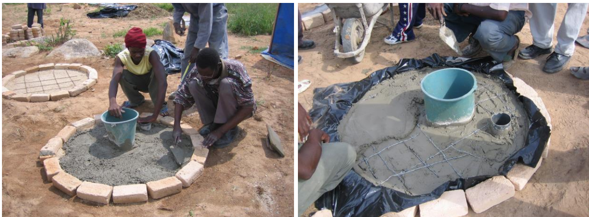
Filling the mould with the concrete mix
