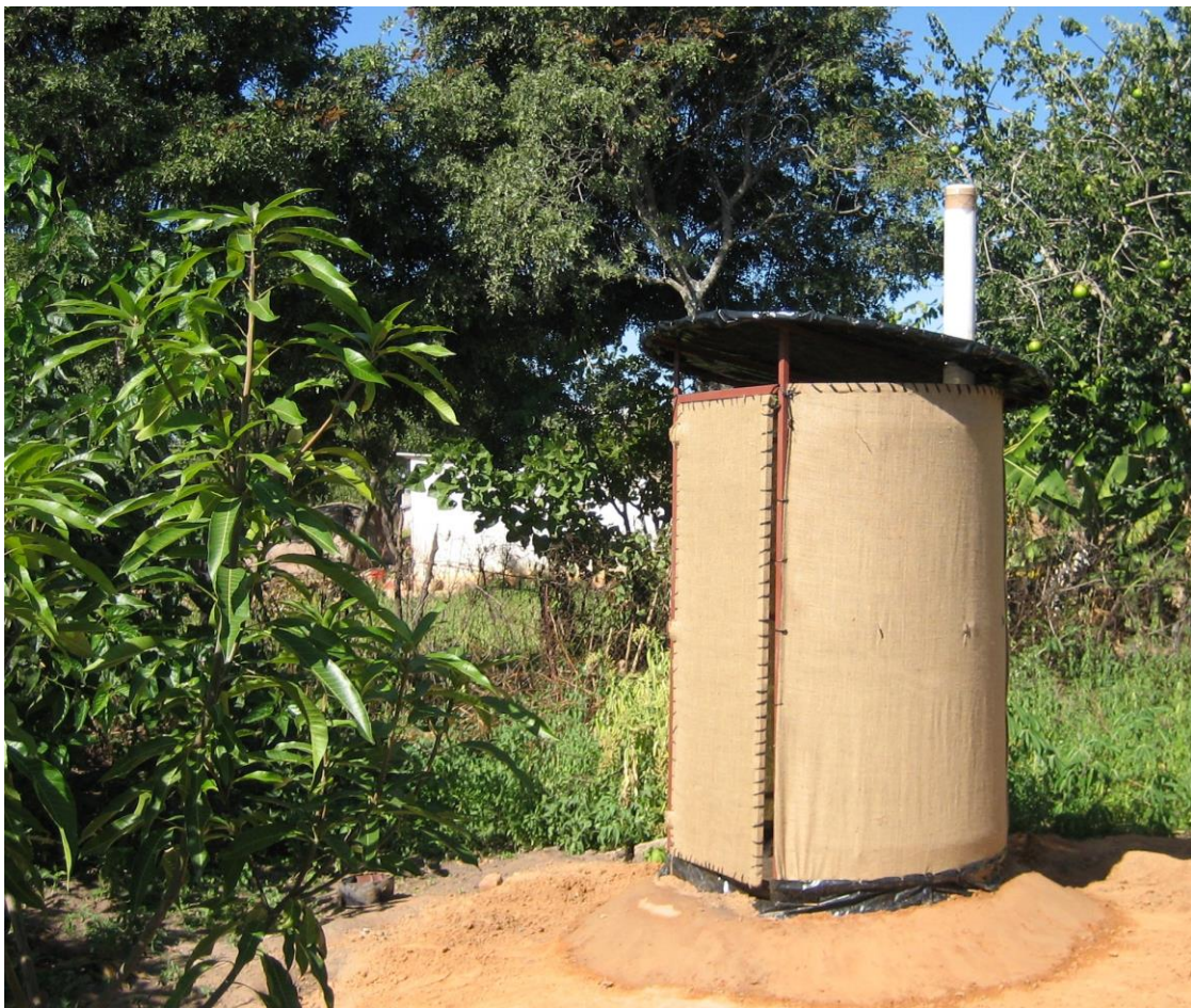
An early ventilated Arborloo with portable superstructure built in Epworth in 2010
