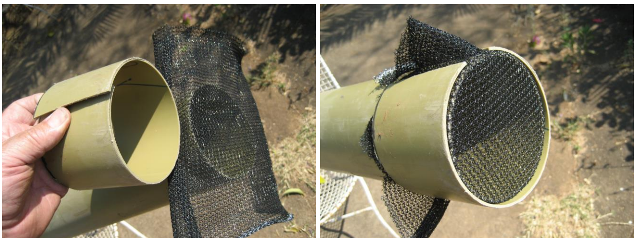
Fitting the fly screen to the vent pipe
