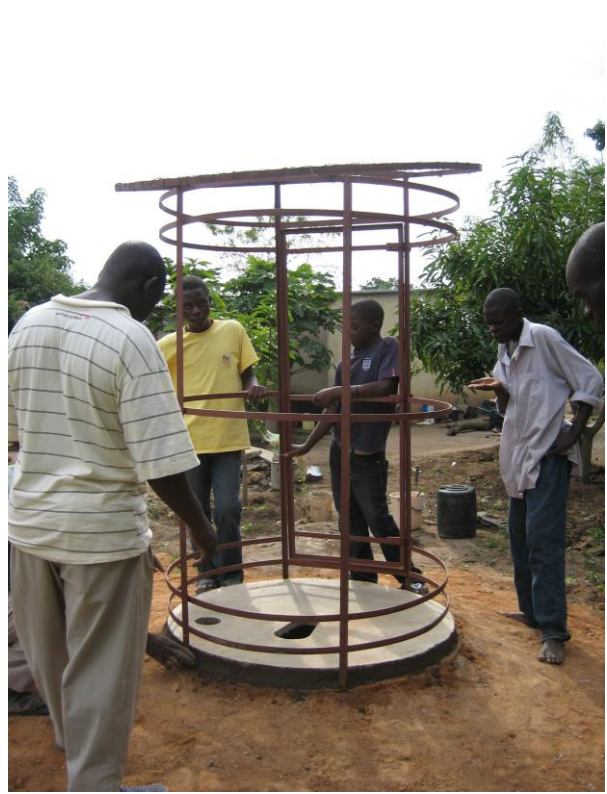
These photos show the design of the steel frame structure, fabricated by V&W Engineering. It is light and strong enough to be carried by 4 people. Its legs sit on the ring beam surrounding the slab.
