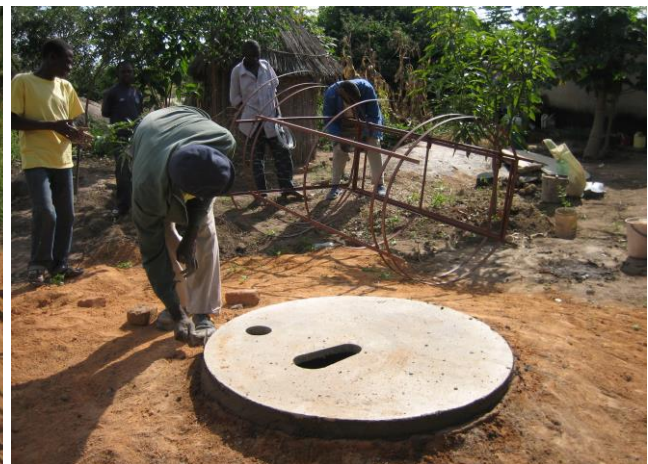
The slab has been placed on top of the ring beam above a pit. In this case a steel framed structure has been used as the following photos show.
