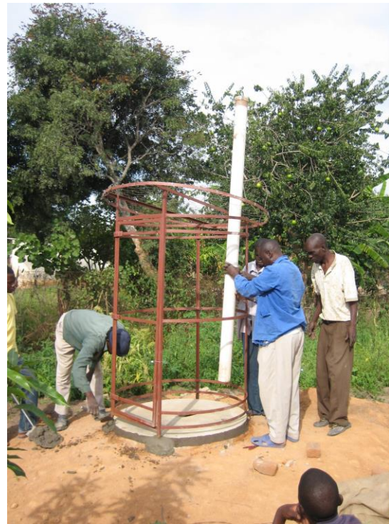
The 110mm PVC vent pipe is being lowered into the vent pipe hole in the slab.
