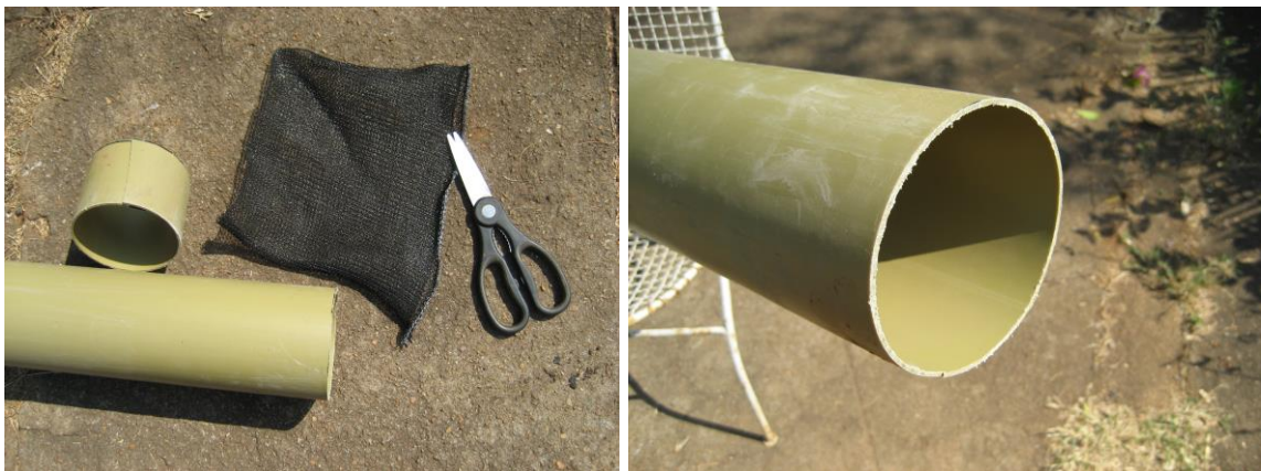
Fitting the fly screen to the vent pipe
