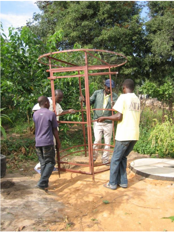
These photos show the design of the steel frame structure, fabricated by V&W Engineering. It is light and strong enough to be carried by 4 people. Its legs sit on the ring beam surrounding the slab.
