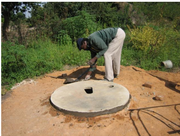
The slab has been placed on top of the ring beam above a pit. In this case a steel framed structure has been used as the following photos show.
