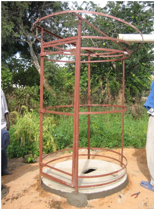
The 110mm PVC vent pipe is being lowered into the vent pipe hole in the slab.
