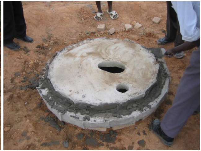
The pit has been dug down. A seal made between the slab and ring beam and the slab levelled. Soil from the pit has been placed around the ring beam.
