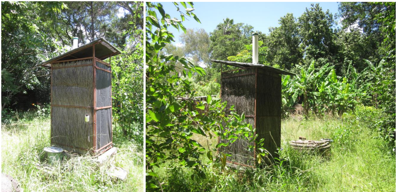
Photos of a rectangular steel framed portable superstructure lined with dried grass. These units have been in operation for several years and have proved to be very effective and long lasting. In the photos shown above, another ecological unit, called a “Skyloo” using a steel framed superstructure is in use. The slab is rectangular in shape. The steel framed structure has also been used for another ecological toilet called a Fossa alterna . The Fossa alterna in this case uses a rectangular ring beam. Two of these are made near to one another and alternate at yearly intervals. Soil, ash and leaves are added to the pit alongside human excreta. The resulting pit material can be dug out and dug into and mixed with soil in small vegetable gardens.
