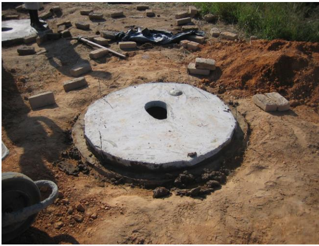
The pit has been dug down. A seal made between the slab and ring beam and the slab levelled. Soil from the pit has been placed around the ring beam.
