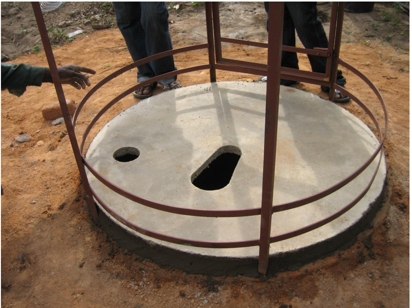
The lower end of the steel framed structure.
