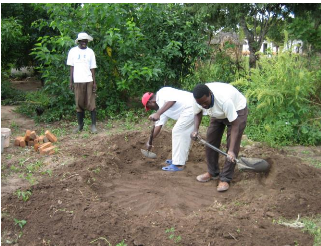
After the site was chosen on slightly raise ground the topsoil was removed and placed to one side. Then a ring was marked on the ground one meter in diameter.
