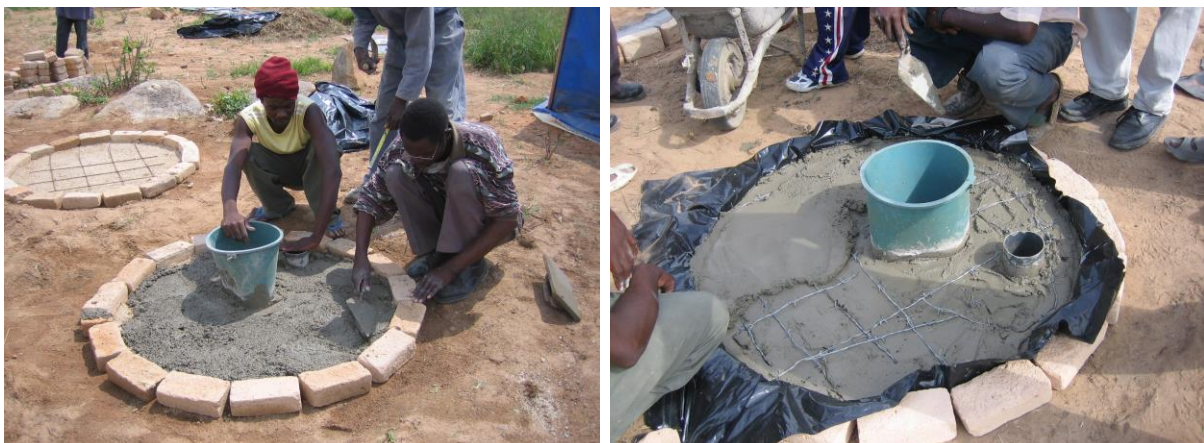
Filling the mould with the concrete mix
