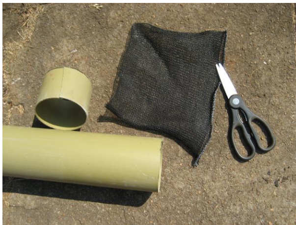
Fitting the fly screen to the vent pipe
