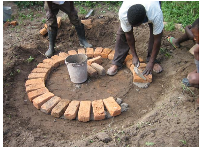
Then a circle of fired bricks was built up bonded with mortar (10:1 mix pit sand and PC 15 cement).
