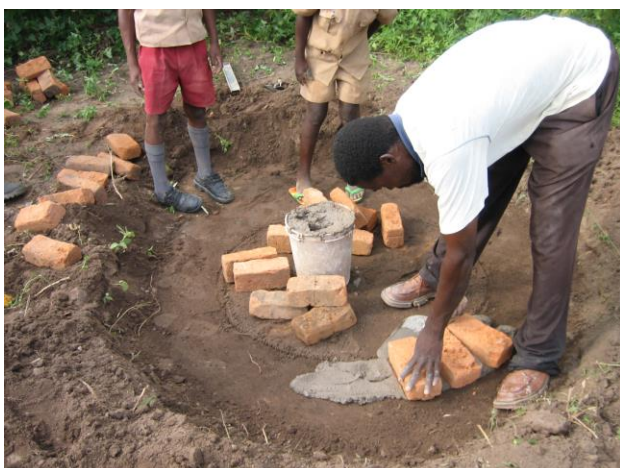
Then a circle of fired bricks was built up bonded with mortar (10:1 mix pit sand and PC 15 cement).
