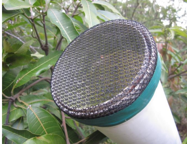
Low cost screen which may be suitable as fly screen on the PVC vent pipe
