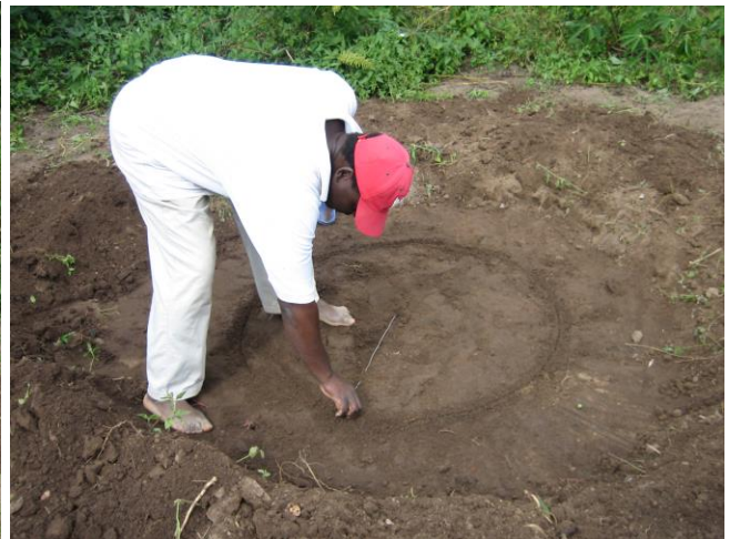
After the site was chosen on slightly raise ground the topsoil was removed and placed to one side. Then a ring was marked on the ground one meter in diameter.
