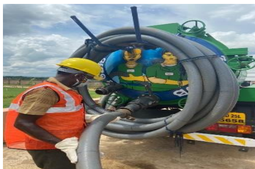
Figure 11: Septic tank emptied by cesspool (Source: Dimple Behal/CSE).
