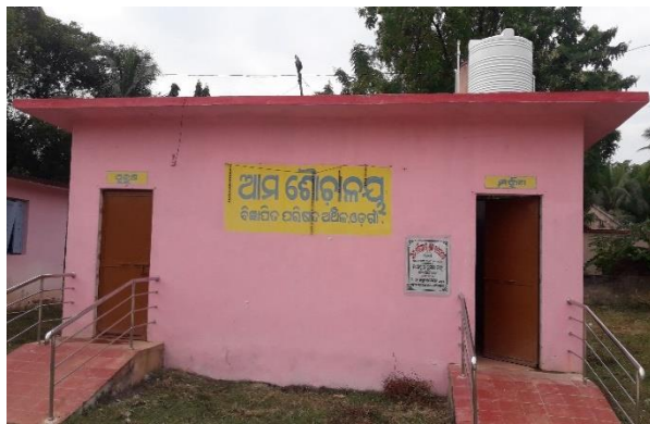
Figure 10: Public Toilet in Odagaon (Source: Dimple Behal/CSE).
