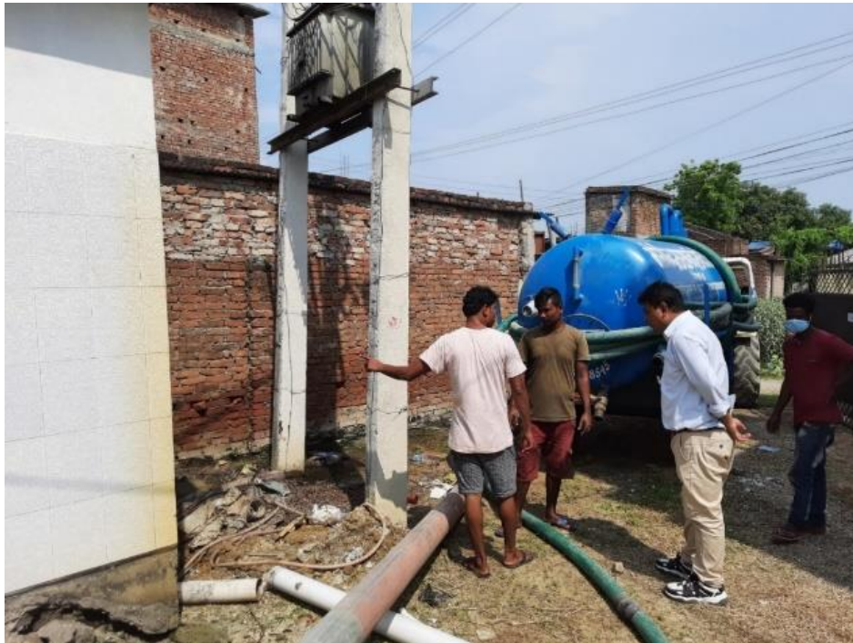
Figure 11: Mechanical emptying of the containment in Siraha Municipality.
