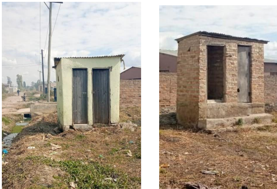
Figure 4: Typical VIP latrines found in Choma Town.
