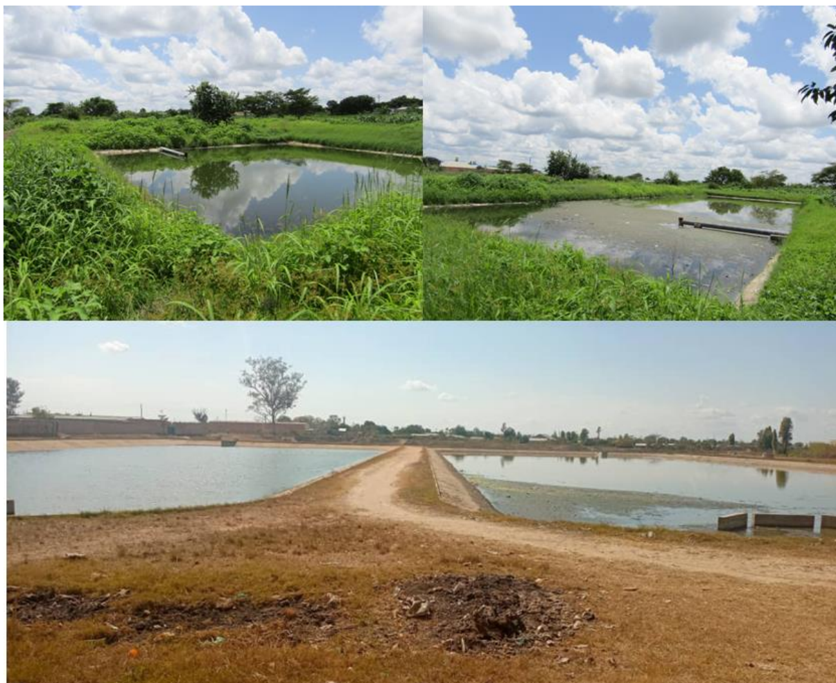
Figure 3: The status of the wastewater stabilization ponds in Choma (Top: The Macha Ponds which need maintenance of the surroundings; Bottom: The well maintained Shampande WWSPs.
