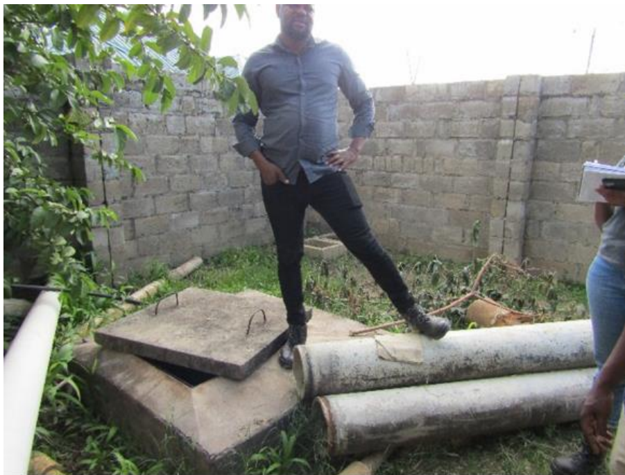
Figure 3: Pollen pimp station currently operating as a communal septic tank (Source: Author).
