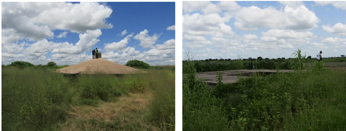
Figure 7: Anaerobic pre-treatment facilities. RHS: an anaerobic tank upstream of the Katondo Ponds; LHS: a septic tank upstream of the Old Ngungu Ponds. (Source: Author).
