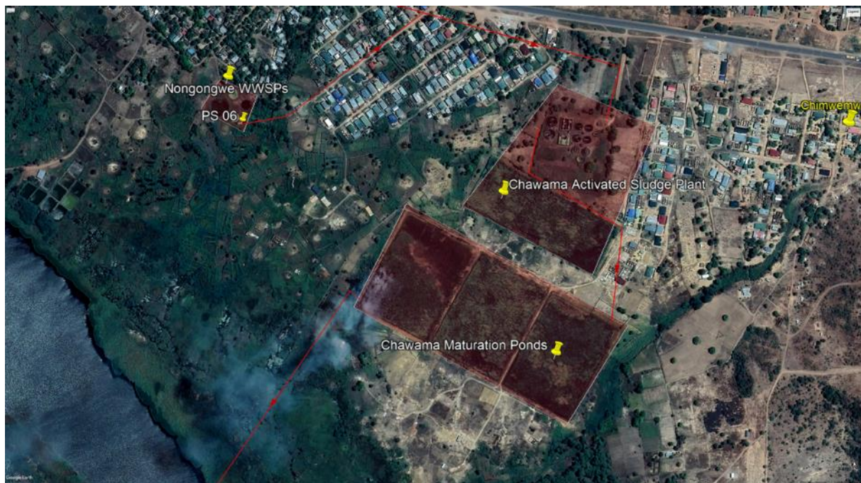
Figure 7: Wastewater Treatment Plants in Kafue.
