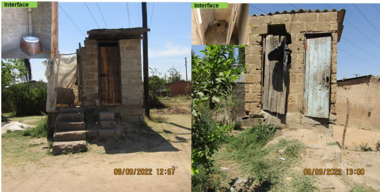
Figure 12: Common type of latrine in Kafue with inserts of examples of user interfaces.
