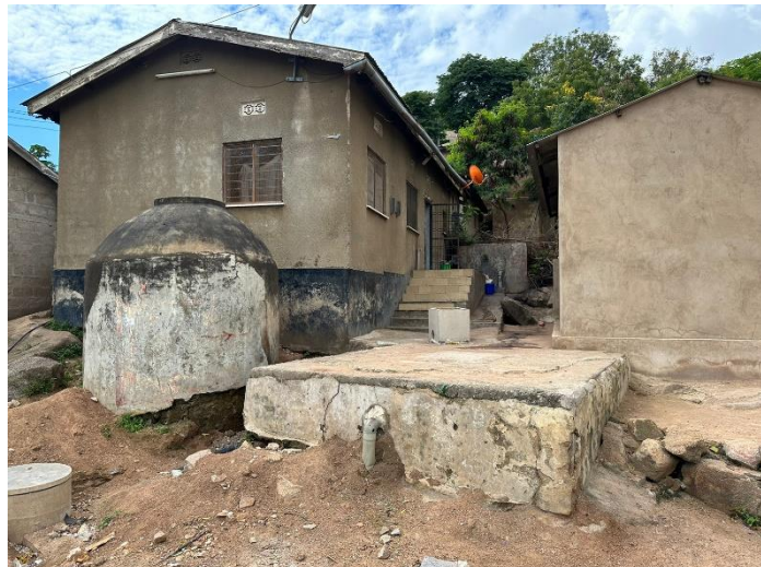
Figure 6: FLT connected to ground, in Ibungilo area where simplified sewer was being laid. (Source: Harsh/CSE/2022).
