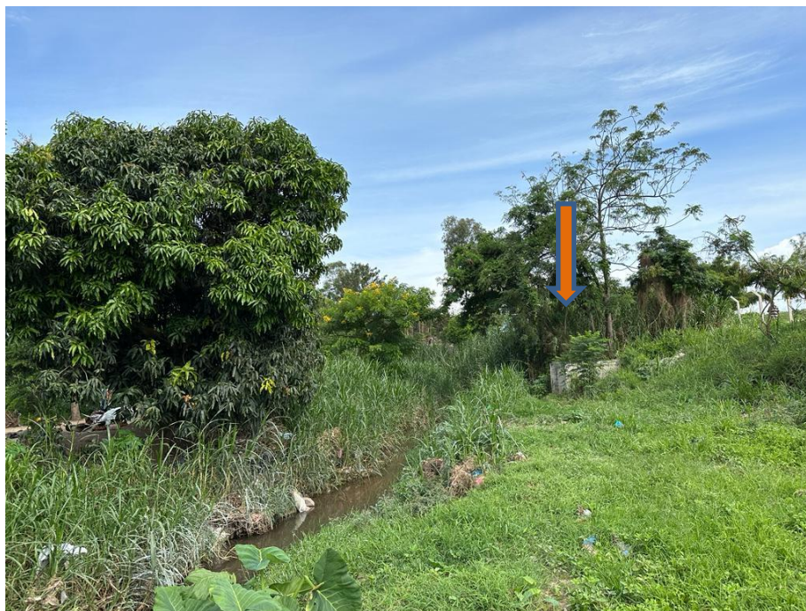
Figure 12: Outlet of WSP (MP6) to stream coming from hills and informal settlements (Source: Harsh/CSE/2022).
