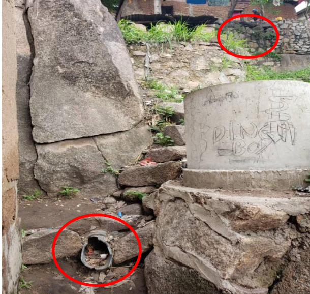
Figure 1: Hidden outlets of Lined tanks with impermeable walls and open bottom. (Source: MWAUWASA).
