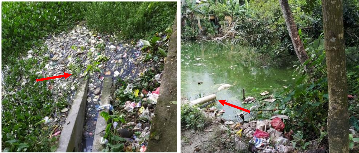
Figure 6: Containment technologies and their connections in Jhenaidah. Left: Septic tank connected to nearby water body, Right: Toilet pipe connected to open environment (Source: Feasibility study 2020-21/DPHE ).
