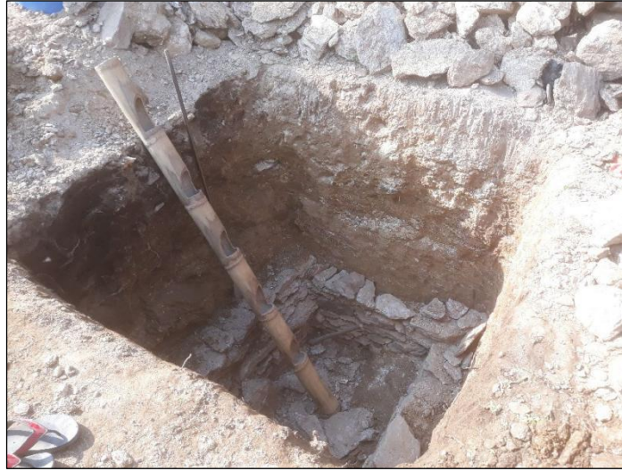
Figure 3: Unlined pit under construction in Ilam Municipality.
