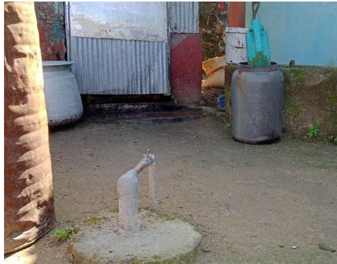
Figure 2: Biogas digester in households.
