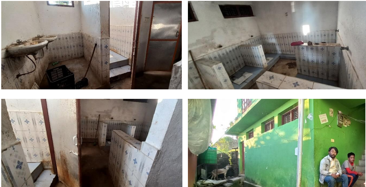
Figure 7: Components of the public toilet at Taxi stand in Ilam Municipality.
