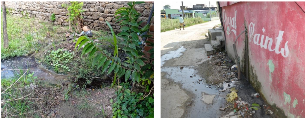
Figure 5: Toilet discharges directly to open environment (left) and open drain (right).
