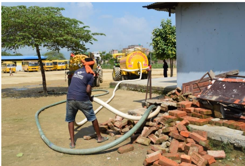
Figure 14: Private desludger emptying containment of a school at Mirchaiya Municipality.
