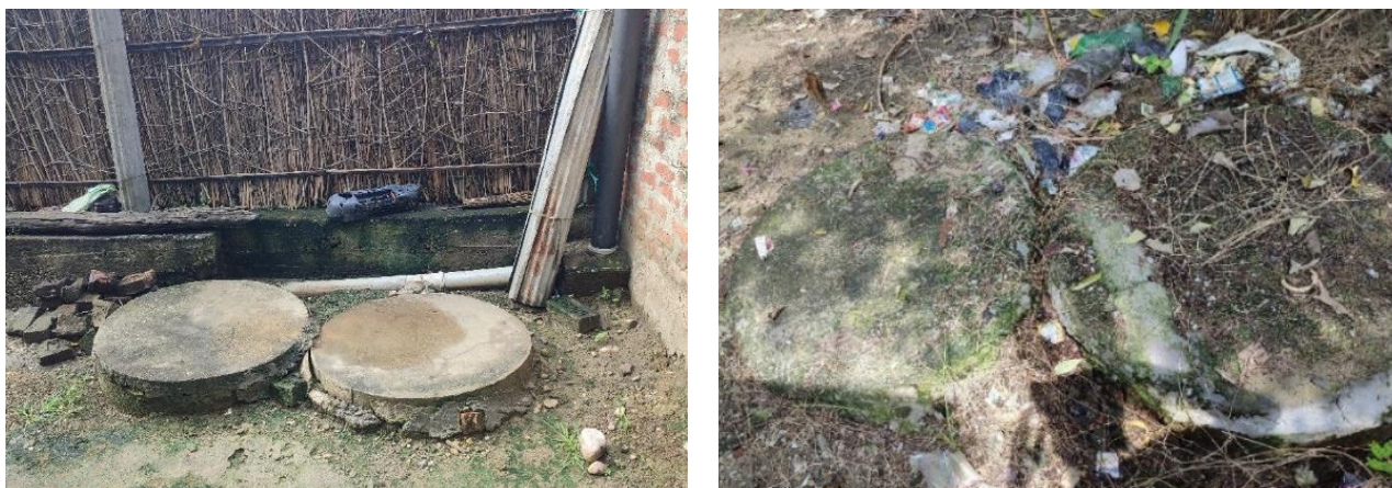
Figure 7: Inappropriate design of twin pits, the distance between two pits is less than 1.2m.
