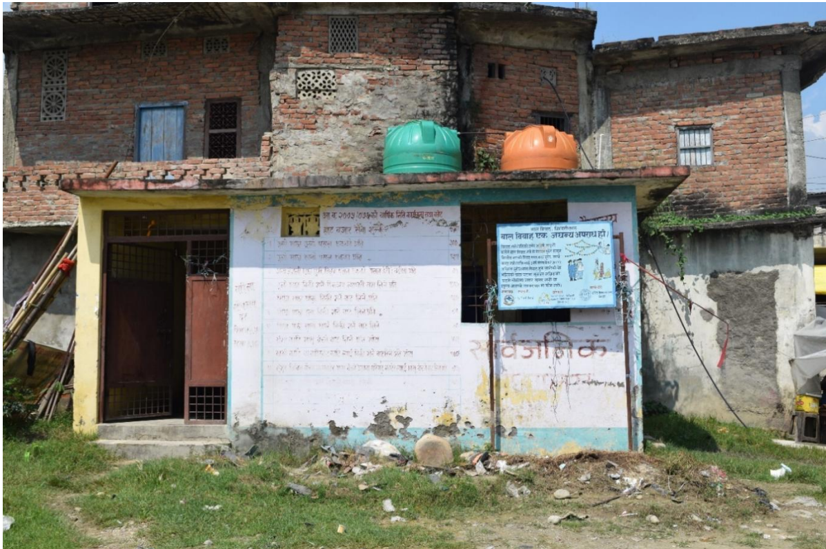
Figure 10: Structure of the public toilet at Mirchaiya bazar.
