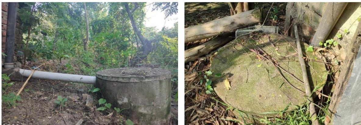
Figure 6: Single pits found in the Mirchaiya Municipality.
