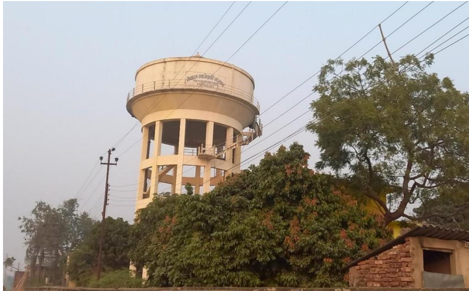
Figure 9: RVT operated by NWSC, Jaleshwar branch.
