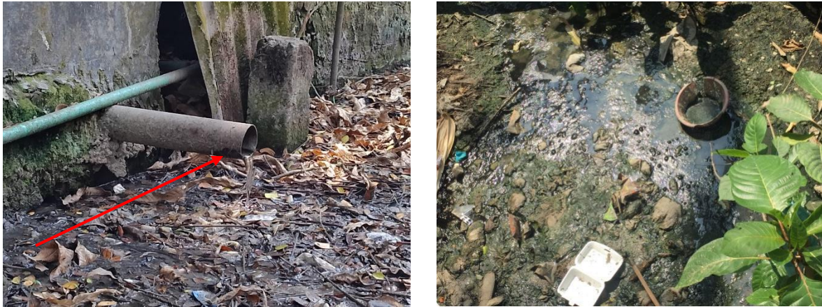
Figure 6: Containment technologies and their connections in Galachipa Municipality. (Toilet outlets connected to open drains) (Source: Field Survey 2023/ O.CREEDS_ WaterAid Bangladesh).
