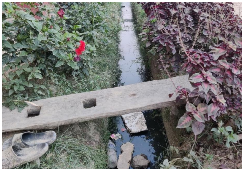
Figure 5: Wastewater in an open drain.
