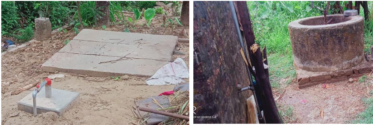
Figure 6: Types of biogas digesters in Sunwal Municipality.
