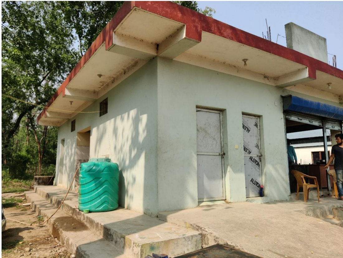
Figure 13: Public toilet located at Ban Kathi, Ward-5.
