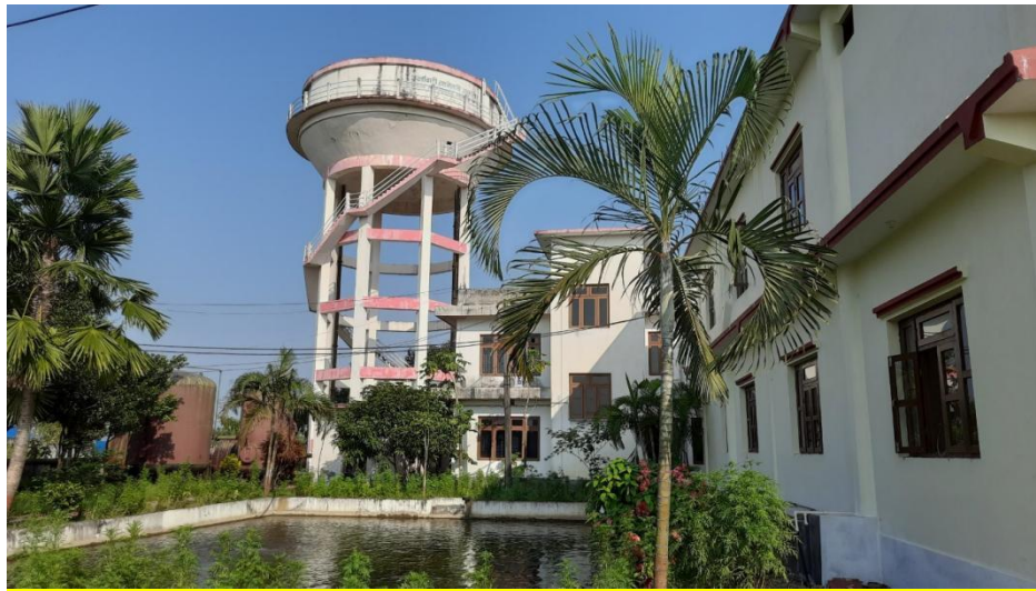
Figure 12: Overhead Tank for Piped Drinking Water Supply System in Urlabari Municipality.
