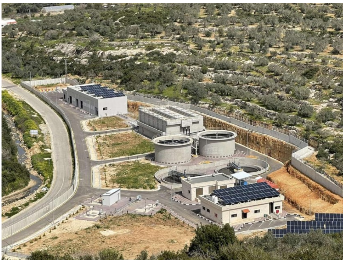
Figure 4: Picture of the WWTP of Salfet City.
