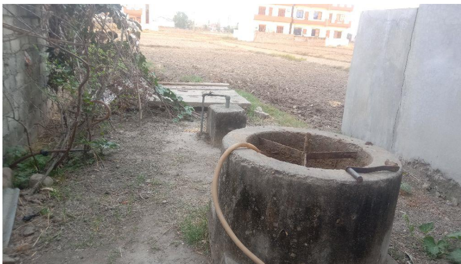
Figure 3: Biogas digester in a household.
