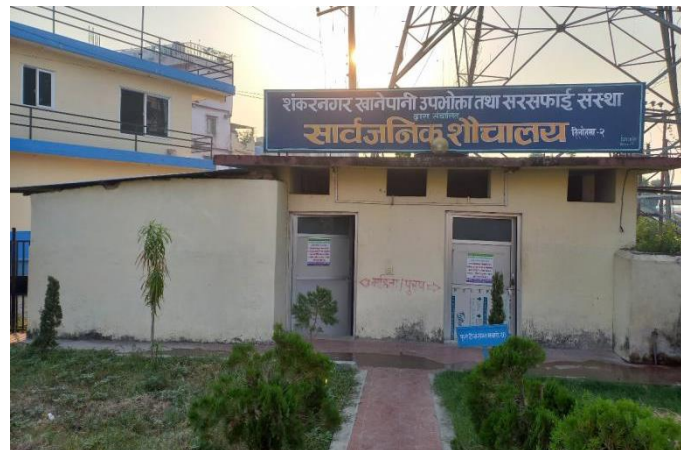
Figure 10: Public toilet in Tilottama Municipality.
