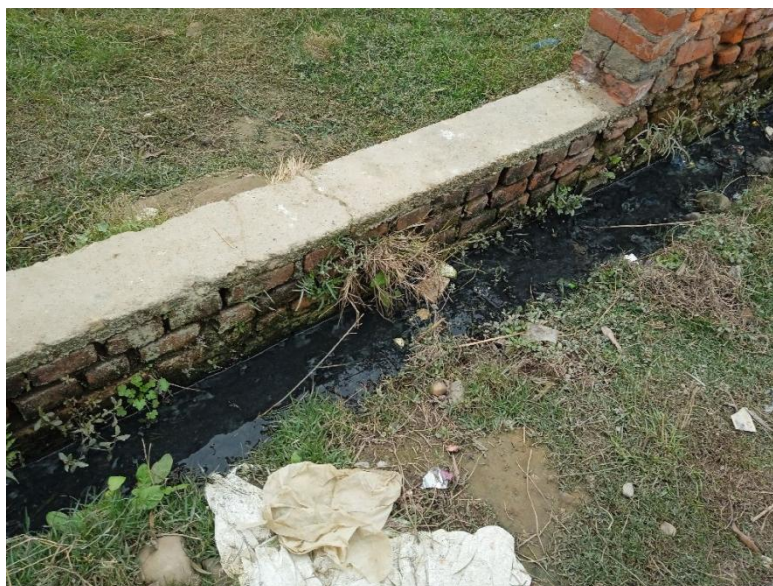
Figure 5: Flow of blackwater in an open drain.
