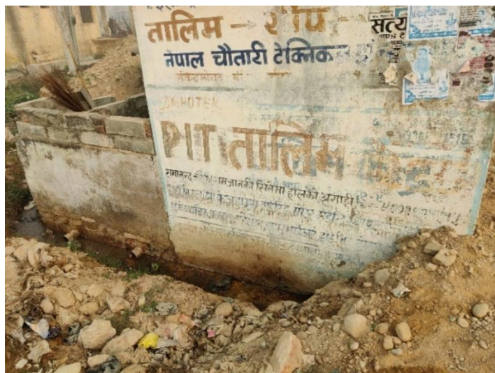
Figure 13: The outlet of the toilet at Pidari Chowk .
