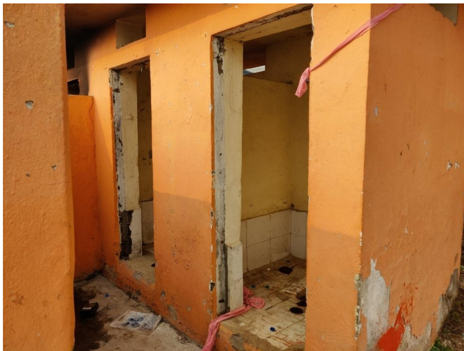
Figure 17: Picture of toilet at Baarah Bigha .
