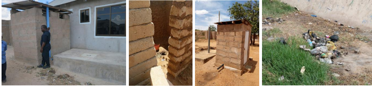
Figure 3 Examples of OSS and “Flying toilets” in Dodoma City Council
