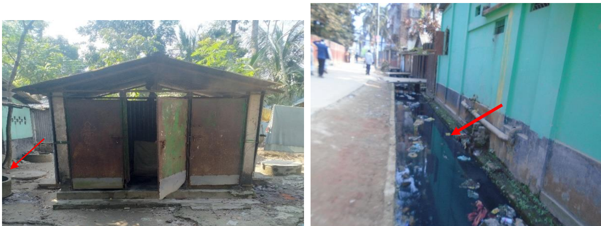
Figure 6: Containment technologies and their connections in Jhalokathi. Left: Toilet Pit open to a nearby water body, Right: Toilet pipe connected to open environment (Source: Feasibility study 2020-21/DPHE ).
